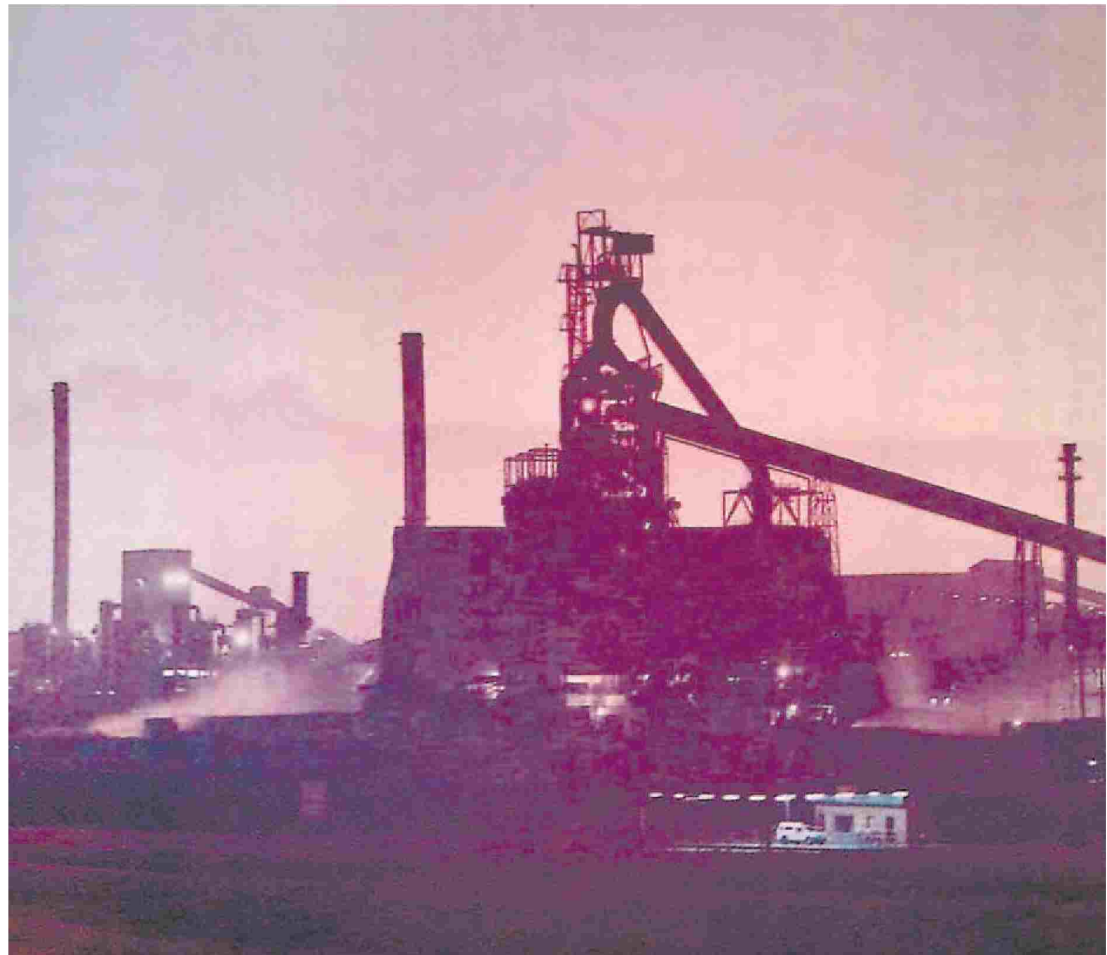
ArcelorMittal will be on shutdown for the next 125 days for a major reline project on the blast furnace.
